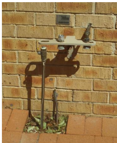
Figure 7.1: Gas is gone – the meter has been removed!
